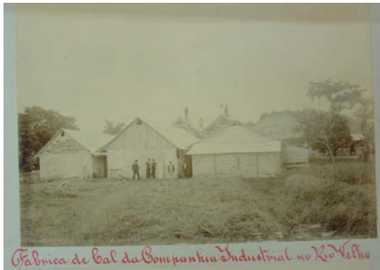
Figure 8 - Lime kilns with ovens and Velho River Shellmound in the background, Joinville/Brazil
