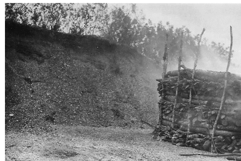
Figure 7 - Lime kiln burning shells in the open air next to Velho River Shellmound, Joinville/SC, Brazil
